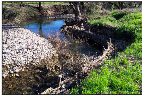
Willow revetment wall along the bank of Selby Creek.
