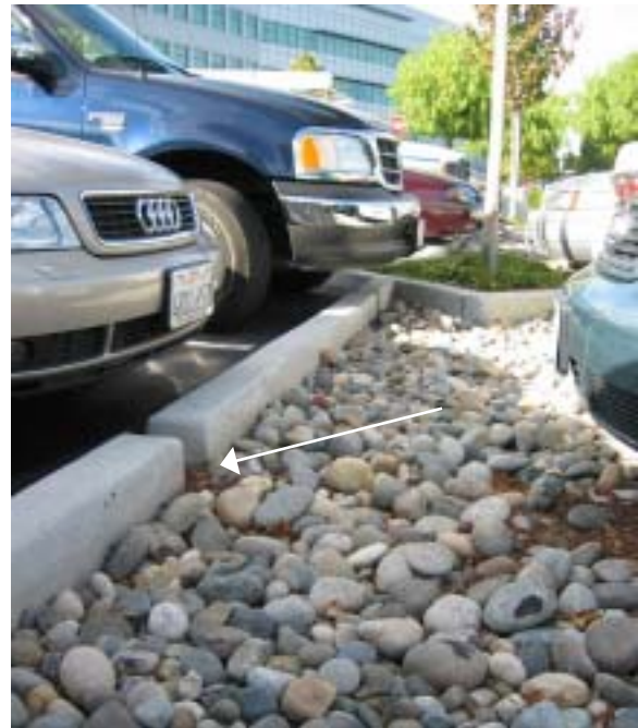
Parking lot runoff drains through curb cuts and then filters through the rocky swale. Trees provide visual amenities as well as reduce the volume and velocity of runoff.
