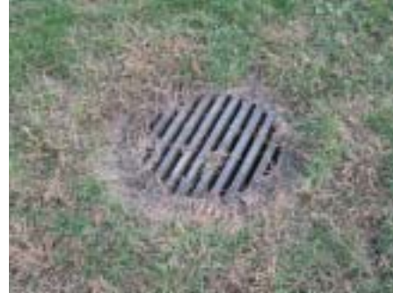
Storm drain shown on the field.
