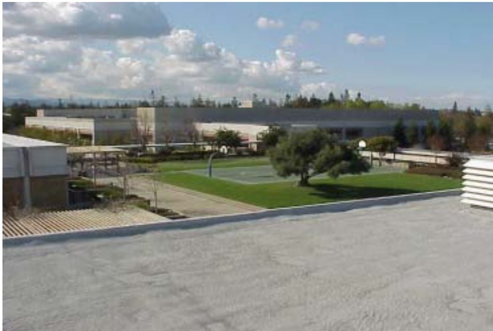
Photograph above courtesy of Scott Sidlow (Agilent)
