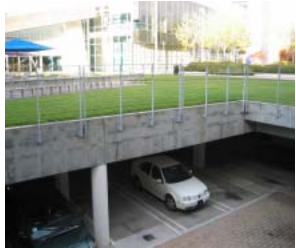
The parking lot can be seen below the turf on the level above.
