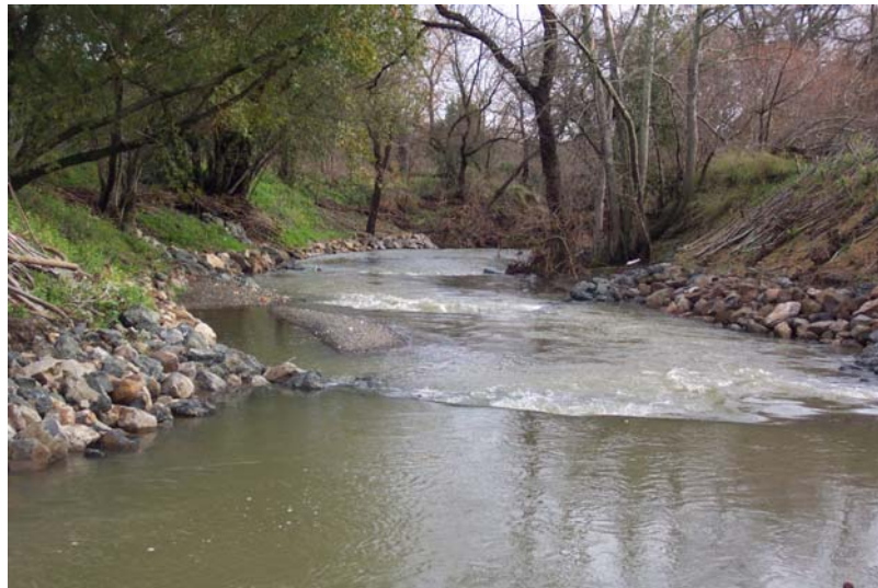
After first rains looking downstream, with all 3 weirs being visible. Note channel thalweg is meandering nicely in the center of channel and fish-passable pools are being scoured in front of the weirs. (January 2008)
