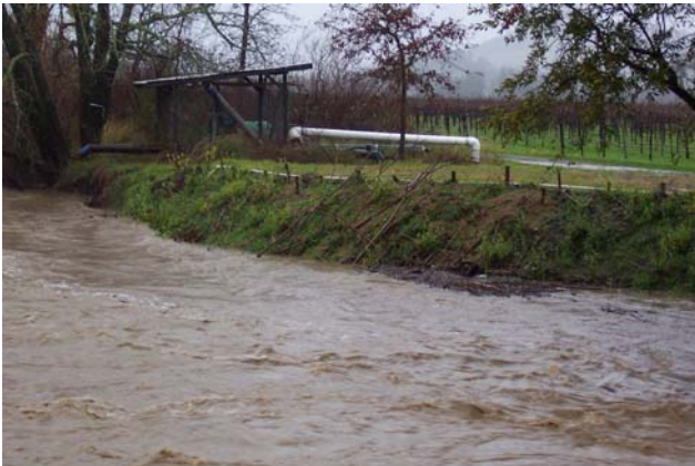
Site observed during first high flows of the season where the water level was just several feet from the top of bank. (January 4, 2008)
