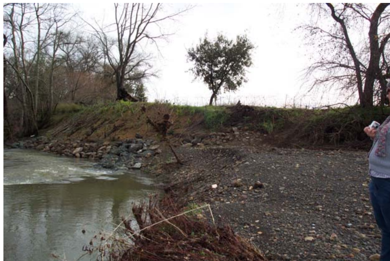
Site observed after flows subsided. Minor erosion of the willow mattress was noted along with variable sediment movement on the gravel bar. (January 8, 2008)
