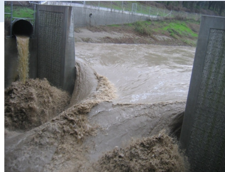
Regional Flood Protection
