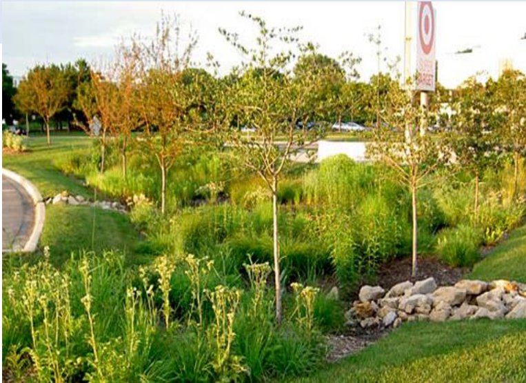
Stormwater Retention and Infiltration
