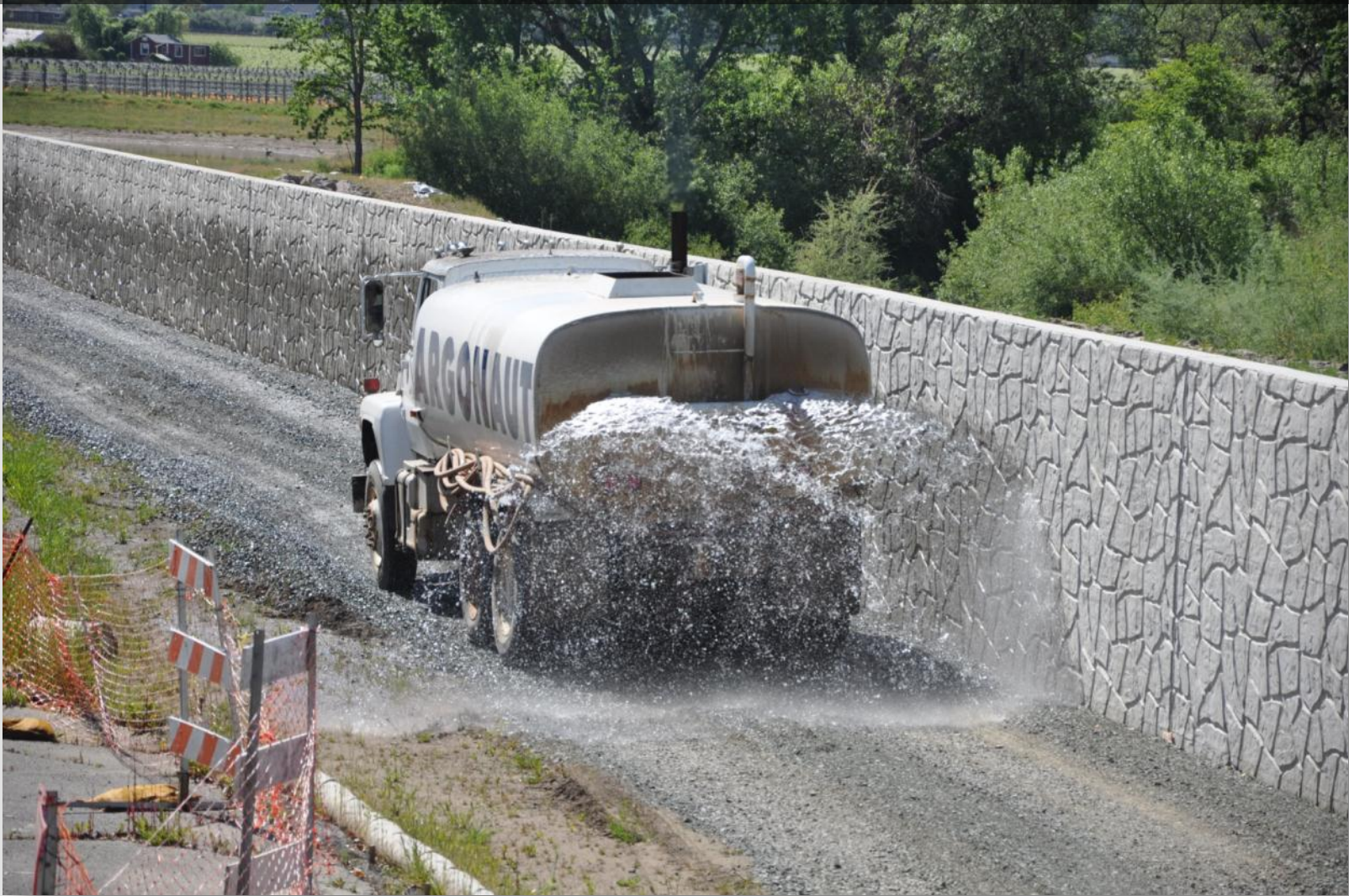
New floodwall during construction
