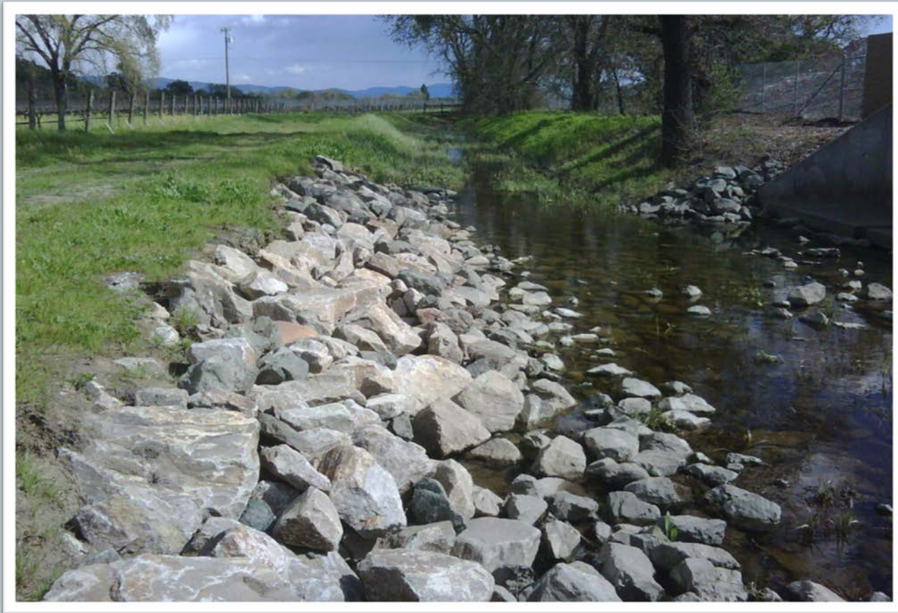
Beard Ditch Bank Repair Completed in 2012
