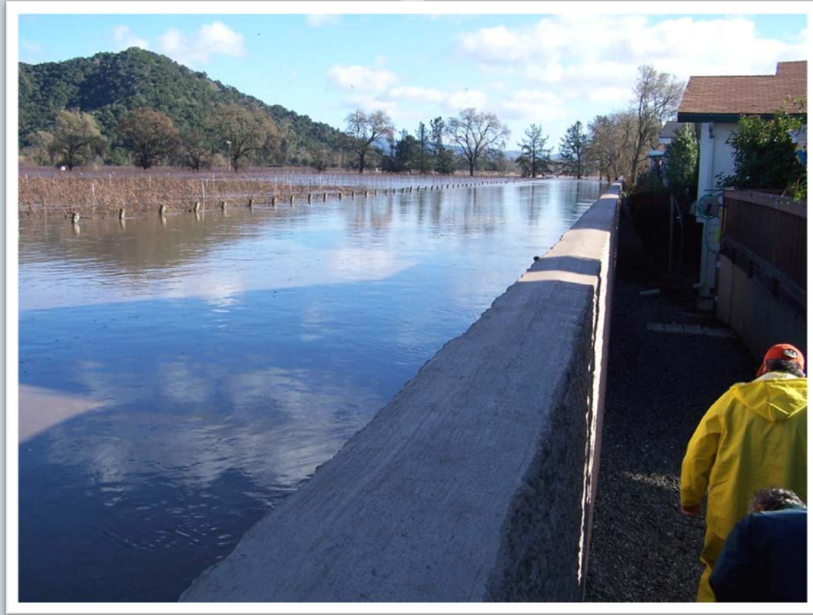
December 2005 flood looking southeast toward Napa River
