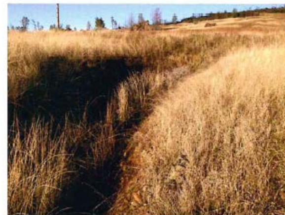
Site 2. Further downstream of the the failed ditch. Restoring historic drainage patterns will prevent further downcutting here.
