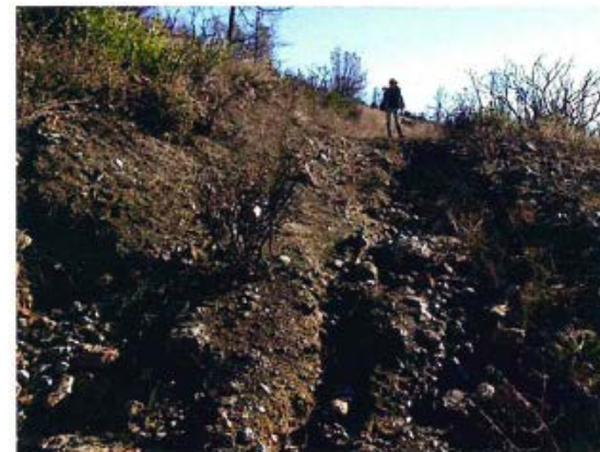
Site 1. One of numerous places along the site 1 road cut where water bars will be built to restore historic drainage patterns.
