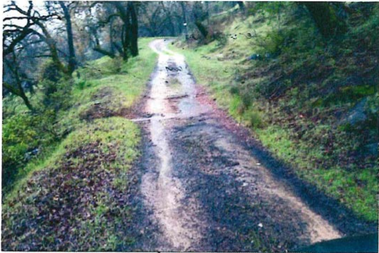
Figure 4. Tire tracks become ditches during rain event.
