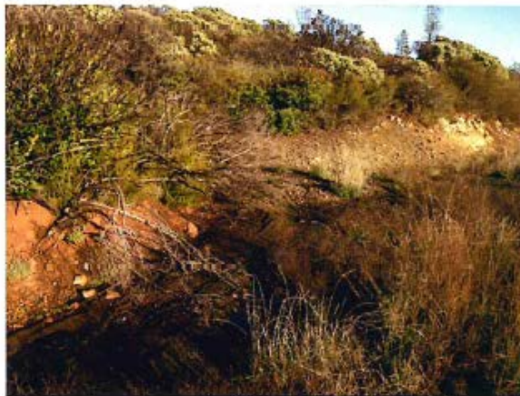
Site 2. The diversion point. Water will be redirected from the ditch, across the right-of-way, into its historic drainage.
