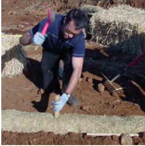
Installation of erosion control
