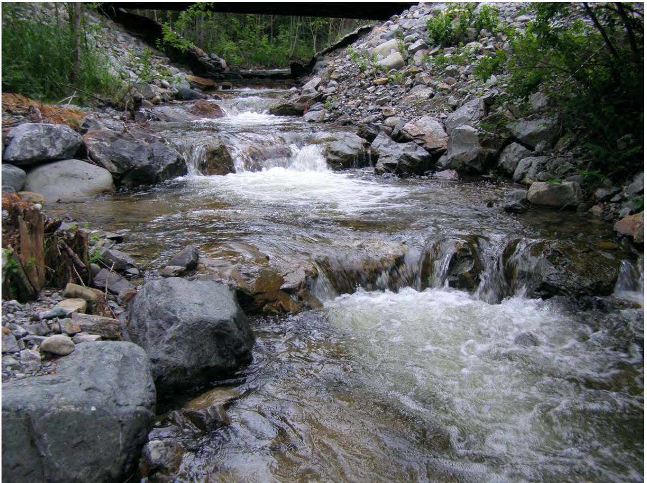
Figure XII-32. Arch-shaped rock weirs produce diverse hydraulics across the crest while concentrating flow towards the channel center. Photo courtesy of Rob Sampson.
