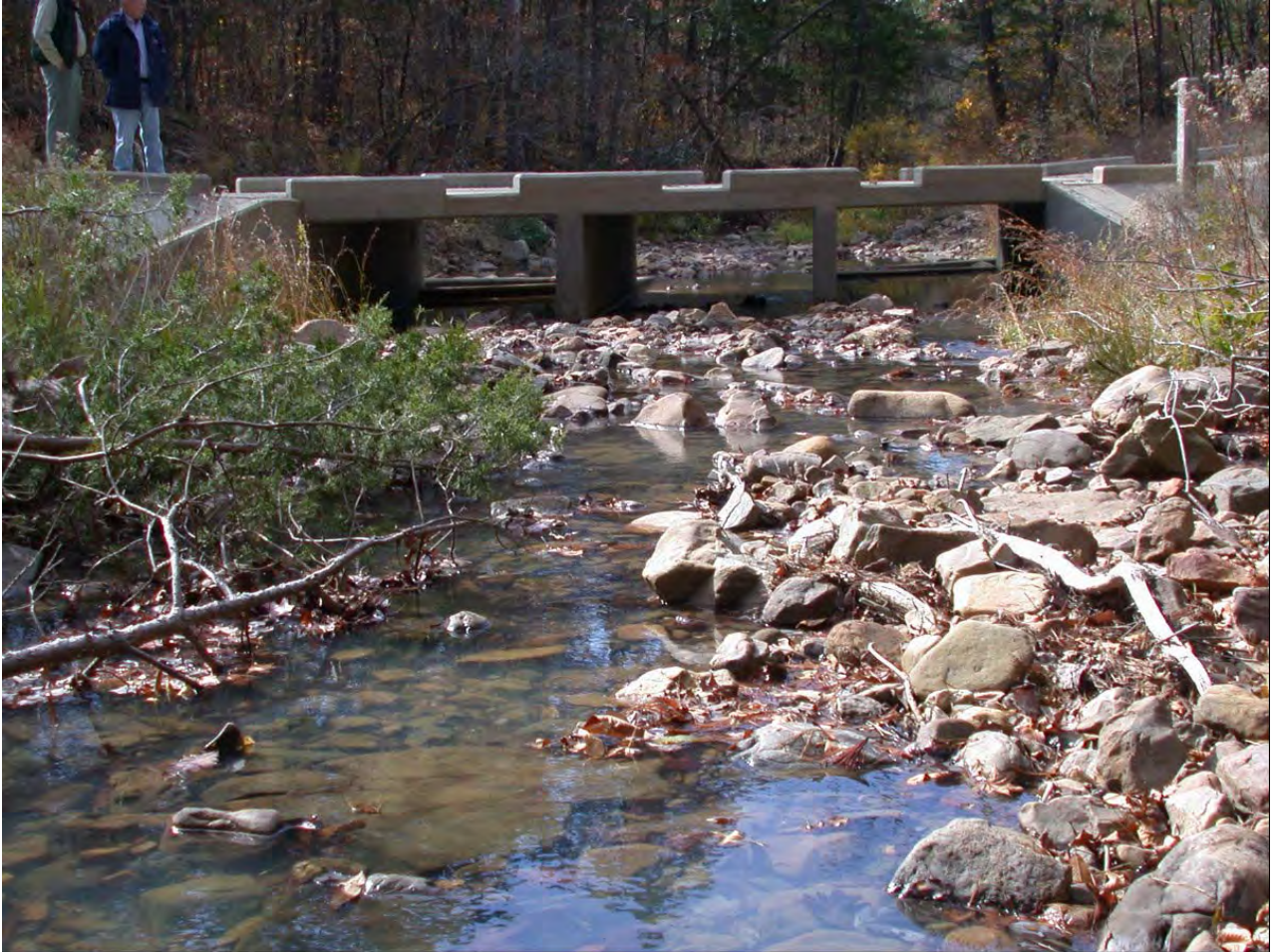
Figure XII-19. A vented ford constructed with three embedded concrete box culverts that span the bankfull channel and convey the bankfull flow without overtopping (FishXing Case Studies 2008).
