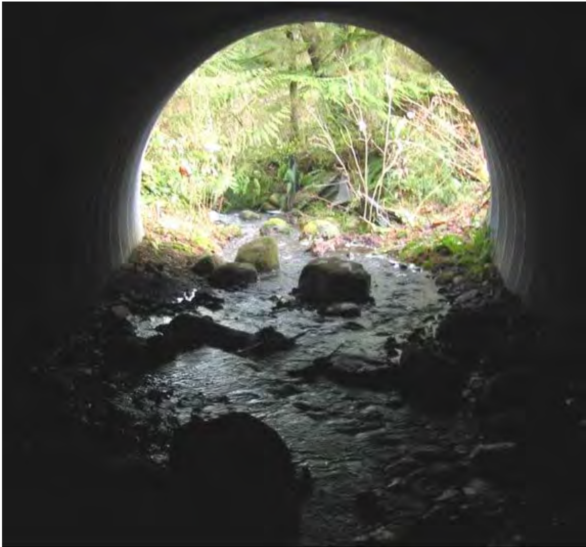
Figure XII-15. Stream simulation channel in Stossel Creek culvert with natural shape, dimensions and key features.
