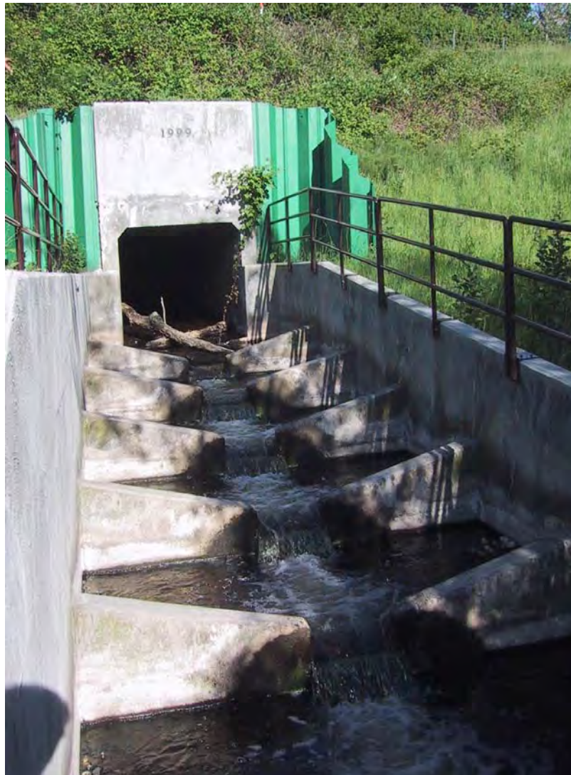
Figure XII-48. Fisher Creek pool-and-chute fishway at low flow.
