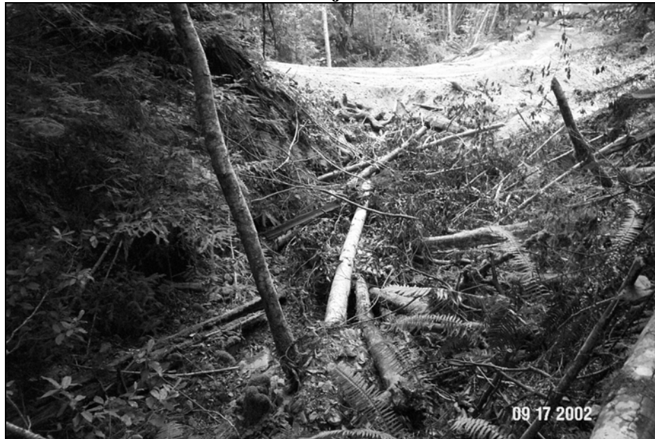
Figure X-D-4. Site #8, 1300 Road, before excavation.
