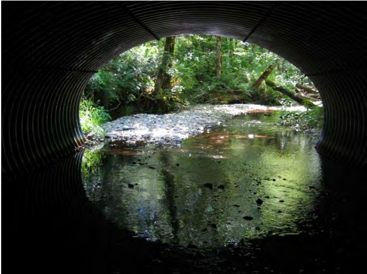
Figure XII-13. Deep Creek. Comparison of diverse bed created by woody vegetation that disrupts the flow and a flat shallow-flow bed within the culvert (Photo: Kozmo Bates).
