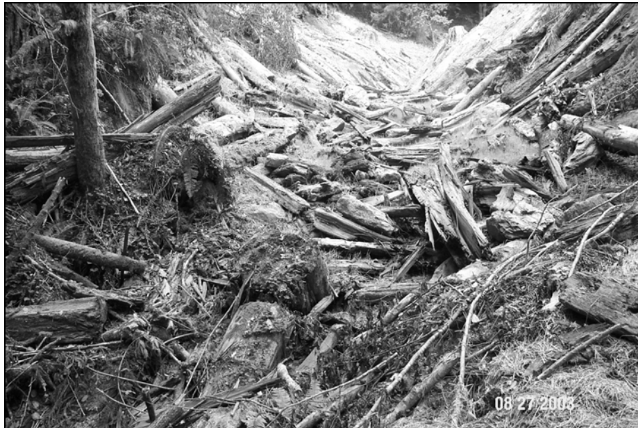
Figure X-D-21. Site # 3, 1311 Road, after excavation. This picture was taken near the same location as the previous photo. The stream crossing has been excavated and an abundance of woody debris has been redistributed along the banks and the channel.
