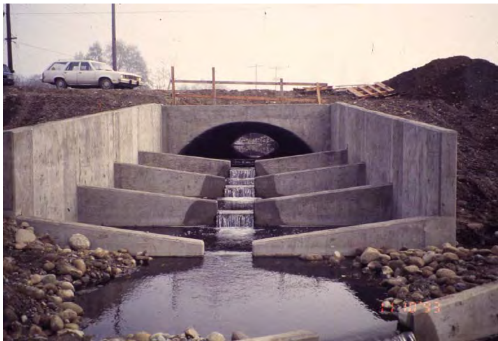
Figure XII-49. Figure Silver Creek pool-and-chute fishway (a) high and (b) low flow.
