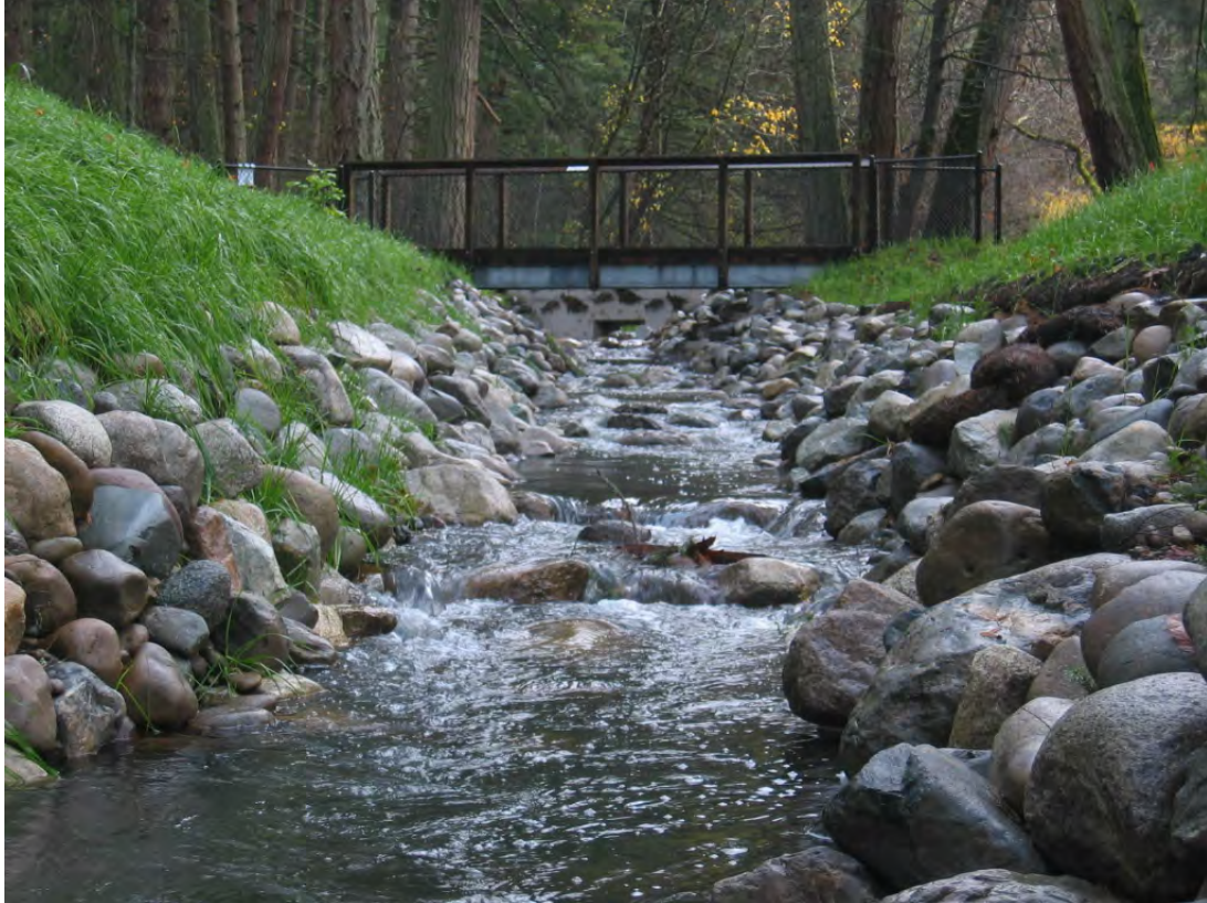
Figure XII-53. Spanaway Creek bypass roughened channel.
