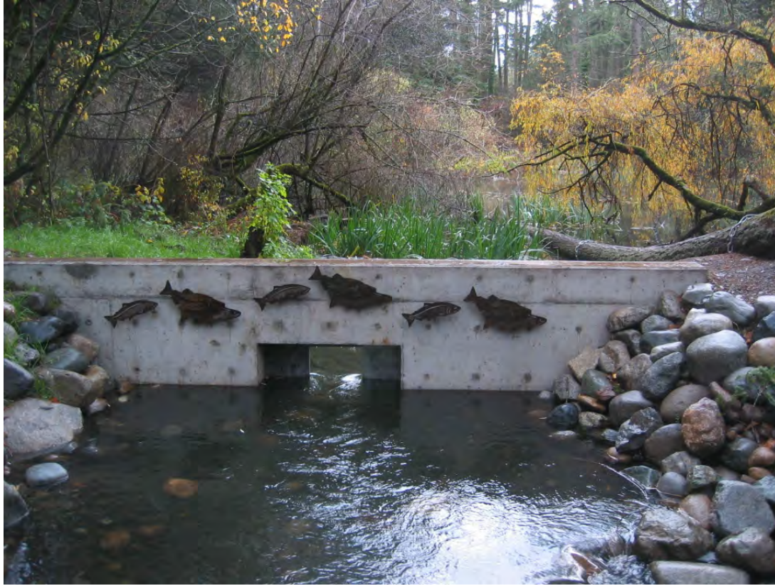
Figure XII-54. Flow control structure, Spanaway Creek bypass channel.
